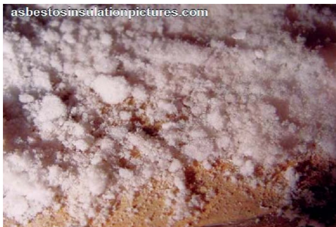
Picture 2. Friable asbestos insulation.
