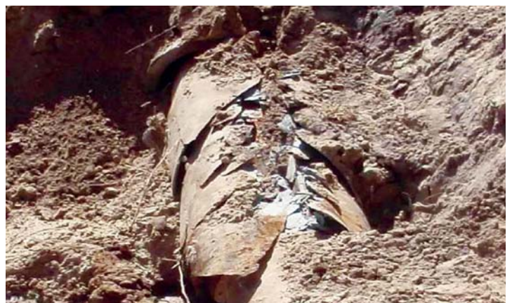
Picture 3. Fractured AC pipe resulting from pipe bursting as it will remain in the ground.
