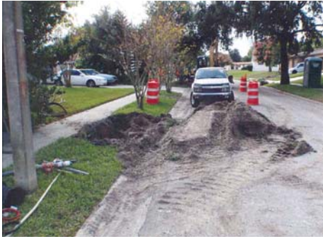
Picture 1. Pipe bursting service connection pit with minimized impact to existing landscaping.
